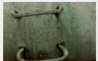
wide view in manholes
