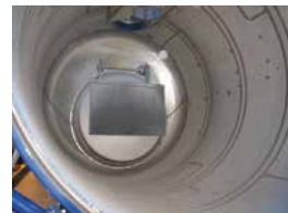
Access filter chamber
