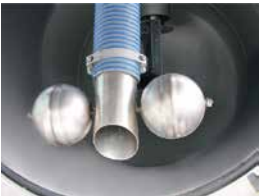
Sludge tank dewatering
